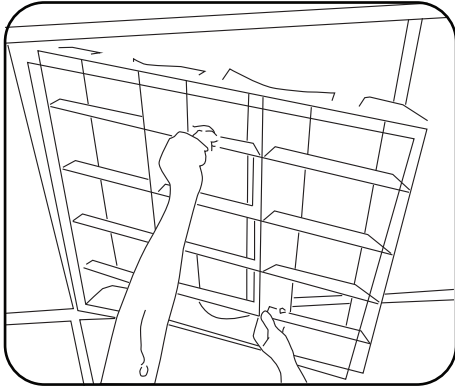
1. Open the cover of the fixture where the magnetic strip kit will be installed.
